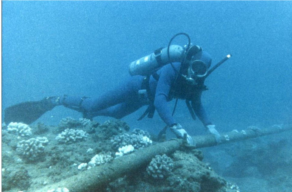
FIGURE 3: “Diver Checking Underwater Protection of Cable” 58
